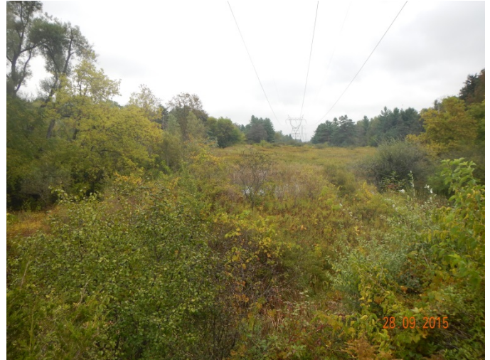
Image 2: View S towards small pond showing roadway along shore.
