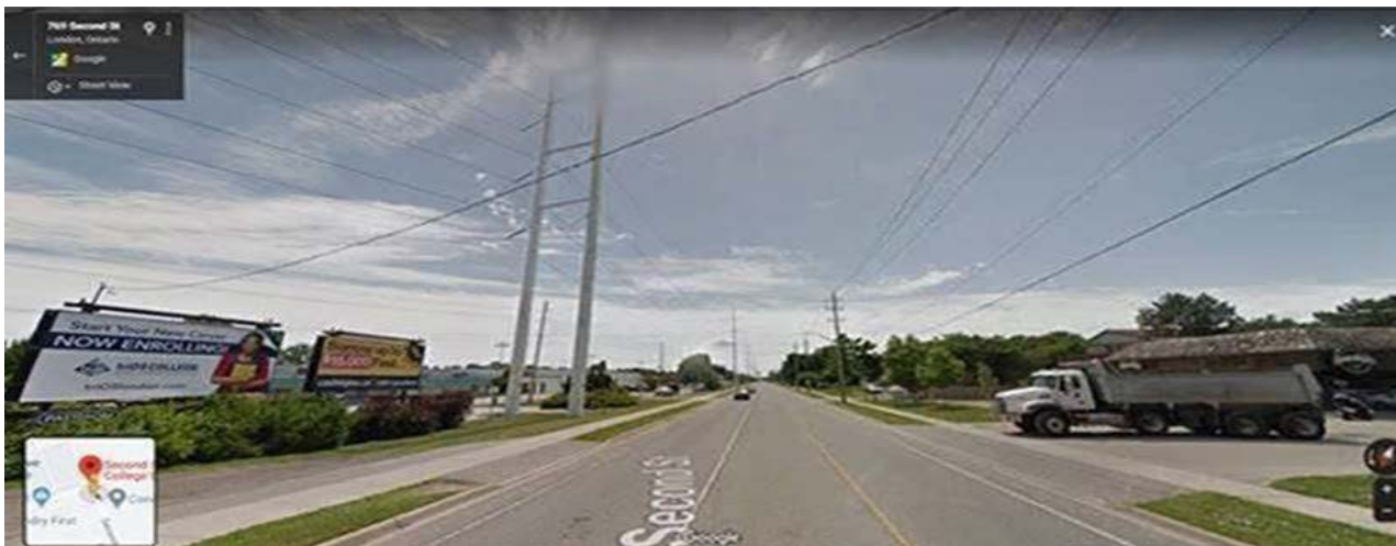
Figure 4 - Steel Tower carrying 230kV double circuits in the city of London – ~1.8km section
