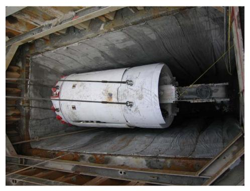
Figure 5 – Example Tunnel Boring Machine
