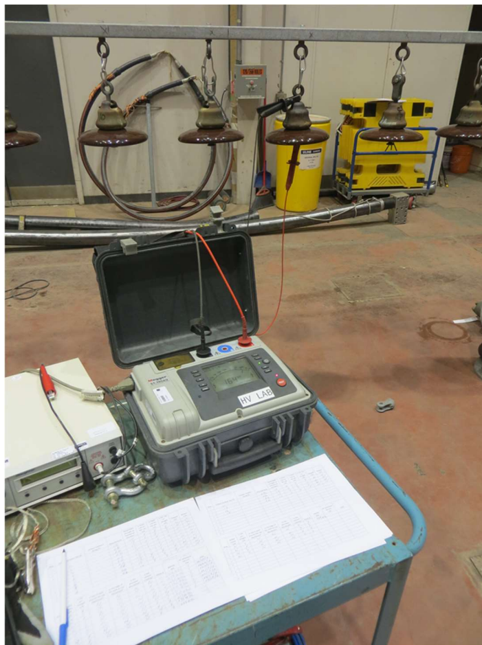
Figure B-2 Insulators undergoing Megger test
