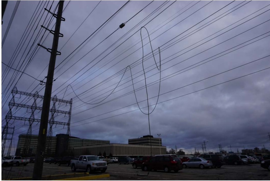
Figure 35 - V76R Insulator Failure
