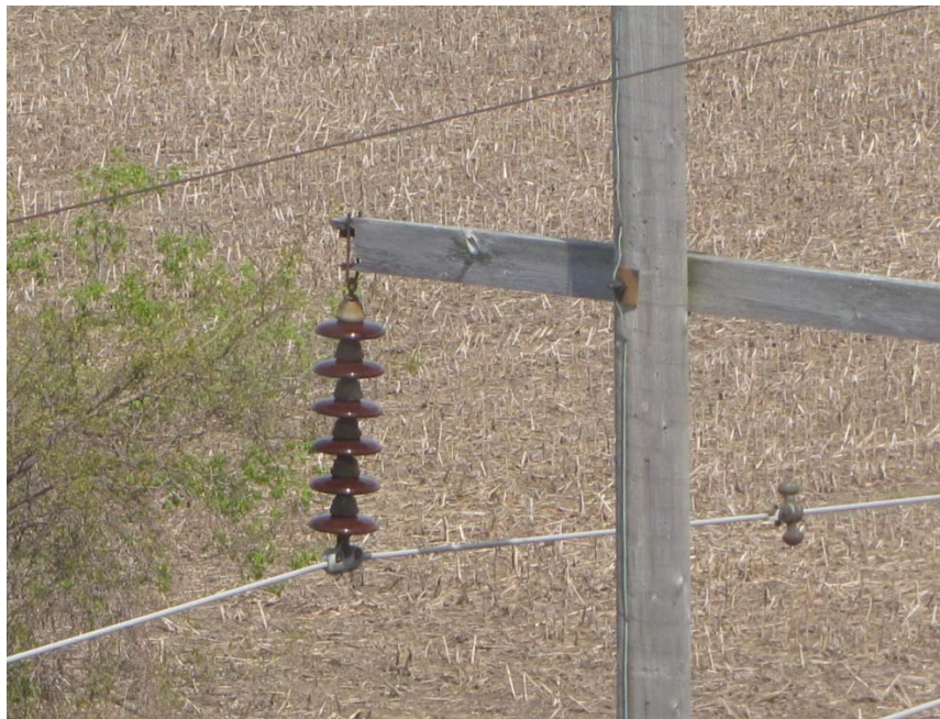
2 Figure 3 – 2017 K2Z (Gosfield Wind CGS x Kingsville TS) wood arm at imminent danger 3 of failure
