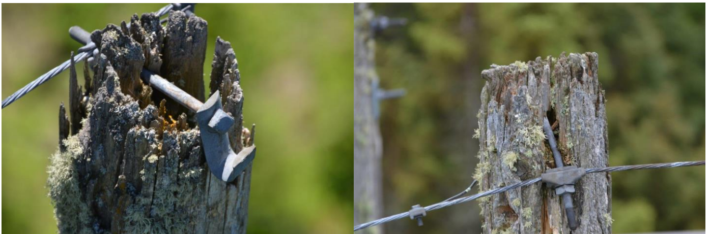
6 Figure 3 - Rotten pole tops on M1T that could fail imminently
