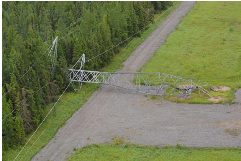
10 Figure 1 - 2016 L20D (Kipling GS x Harmon Jct) steel structure failure due to windstorm
