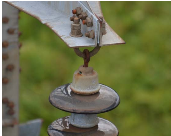
10 Figure 52 - U-bolt on a suspension structure
