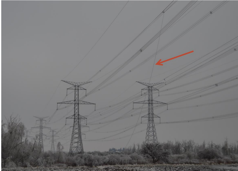
Figure 4 - Fallen span of conductor
