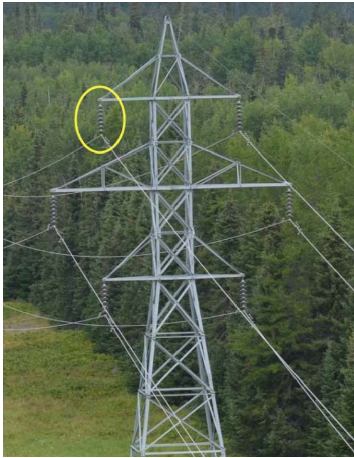
Figure 31 Transmission Line Insulator
